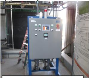
Skid Mounted System Control Panel and Pumps, Tank in Background
