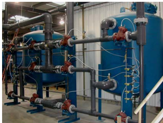
Large dual tank, PLC controlled multimedia filter as manufactured by ProChemTech
